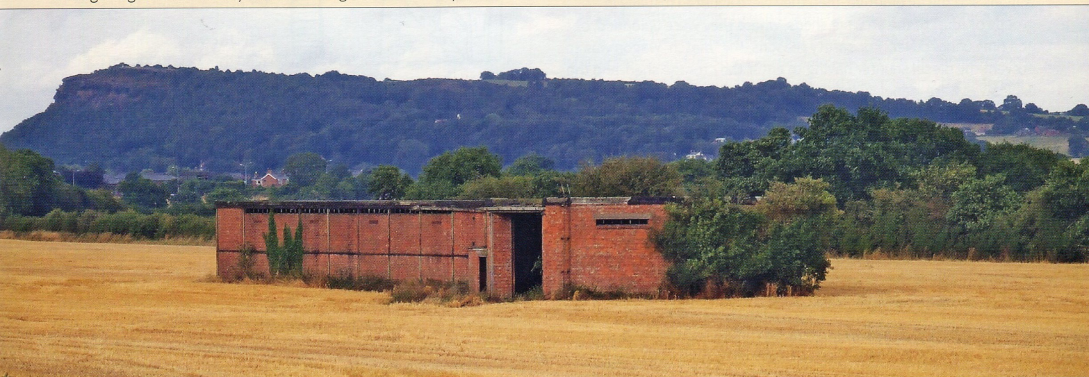
Magazine that has had the surrounding earth mound removed – note the diagonal earth line on the brick blast wall to the right.
