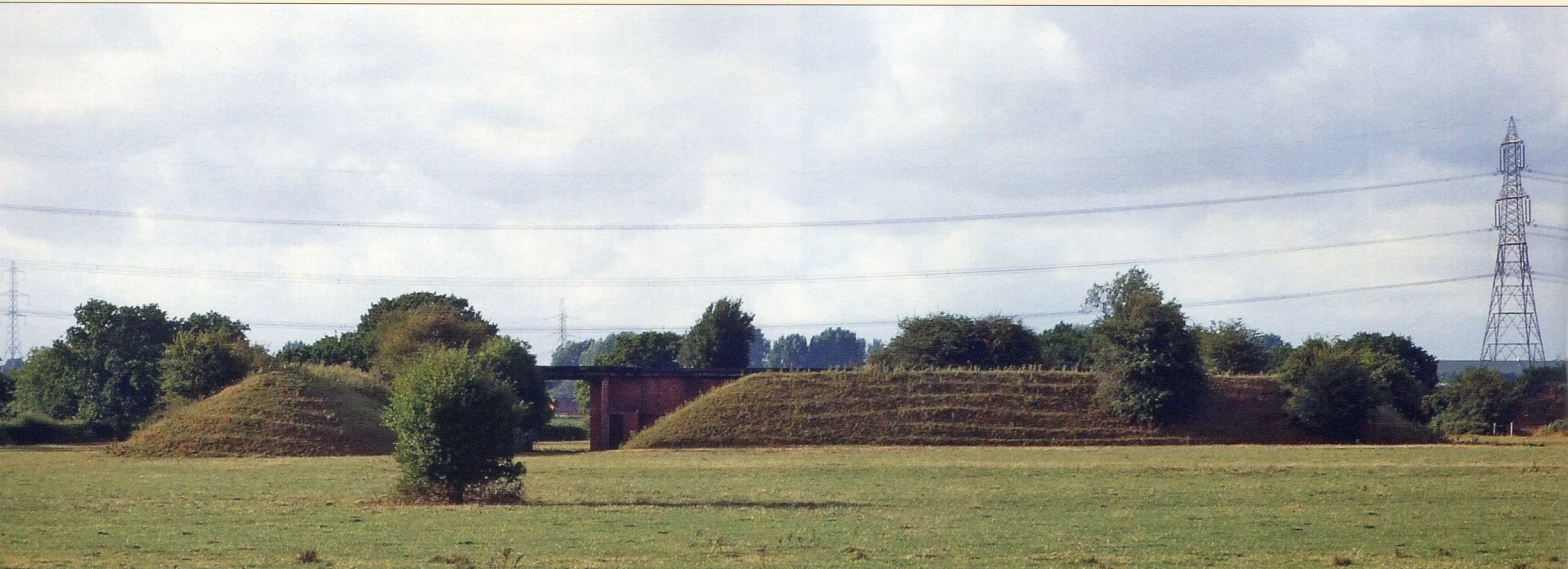
Storage magazine with remaining clay earthworks in a camouflaged design.
