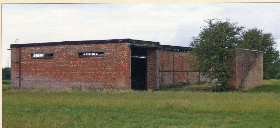
Magazine that has had the surrounding earth mound removed – note the diagonal earth line on the brick blast wall to the right.
