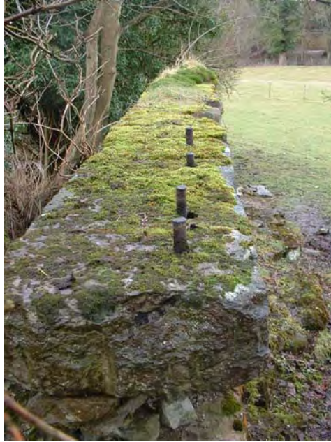
SMR 98057 Detail of reinforcing bars through the eastern elevation of the wheel pit
