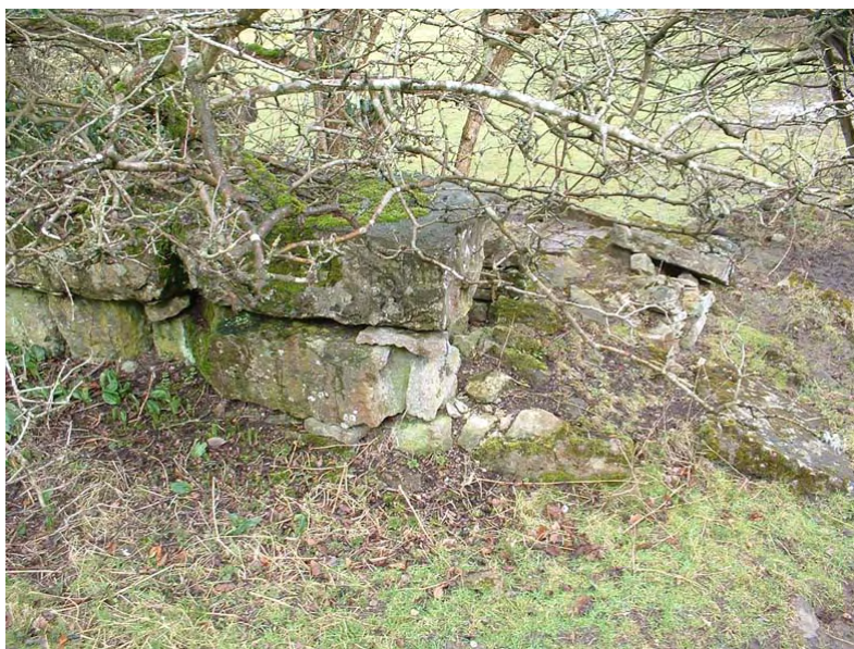
SMR 98057 Detail of external elevation of wheel pit
