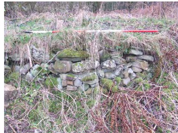
SMR 98059 Detail of the revetment wall for the terrace
