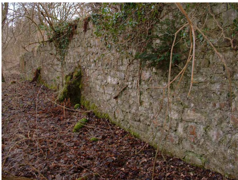
SMR 98049 Internal wall of foundry building with later buttresses
